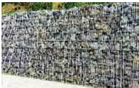
A Gabion kőfal
