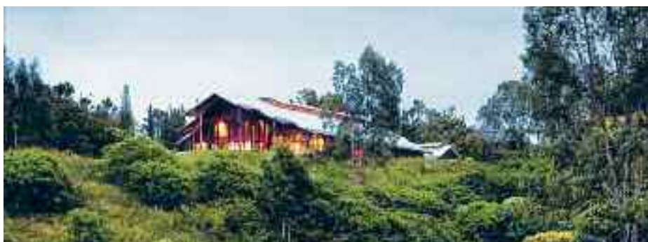
Fotók: Courtesy of Flansburgh Architects
