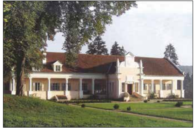
■ Foto 14. Mălâncrav, Conac Apafi, exterior după restaurare © MET ■ Photo 14. Mălâncrav, Apafi Manor, exterior after conservation © MET
