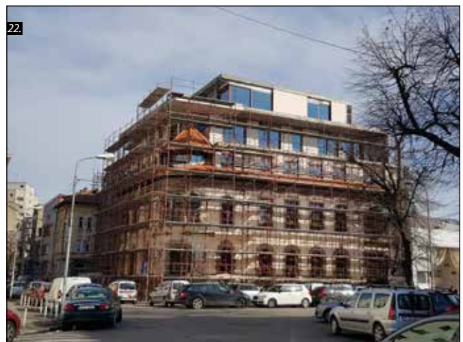
■ Photo 20-22. Bucharest, Dumbrava Roșie Street (protected area no. 40). Well-preserved, neo-Romanian villa, demolished [photo 20, image captured in July 2014 © 2020 Google] while preserving its elevations integrated into a large real estate development © Rodica CRIȘAN 2019, 2020
