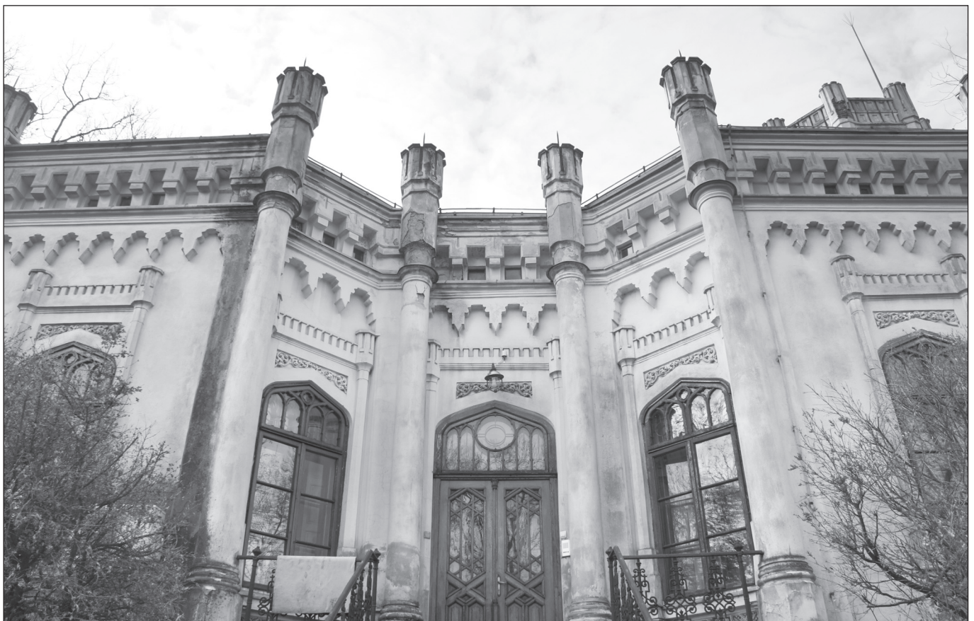
■ Foto 5. Accesul principal ■ Photo 5. Main access
