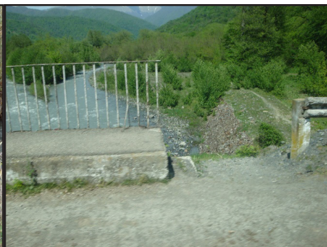
Figure 3. Field survey, Alazani river (project documentation)
