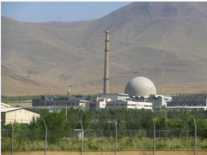
Arak IR-40 Heavy Water Reactor, Iran. Photo: Wikimedia Commons
