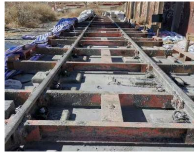
)b) Concrete maintenance of ballastless track
