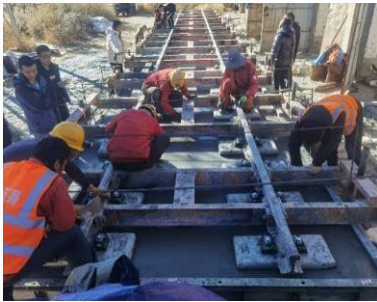
)a) Concrete pouring of ballastless track
