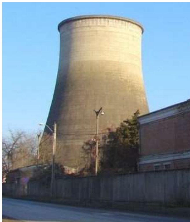
Figure 4: The hyperboloid with a canvas (hyperboloid of rotation). It is a ruled surface with zero Gauss curvature.
