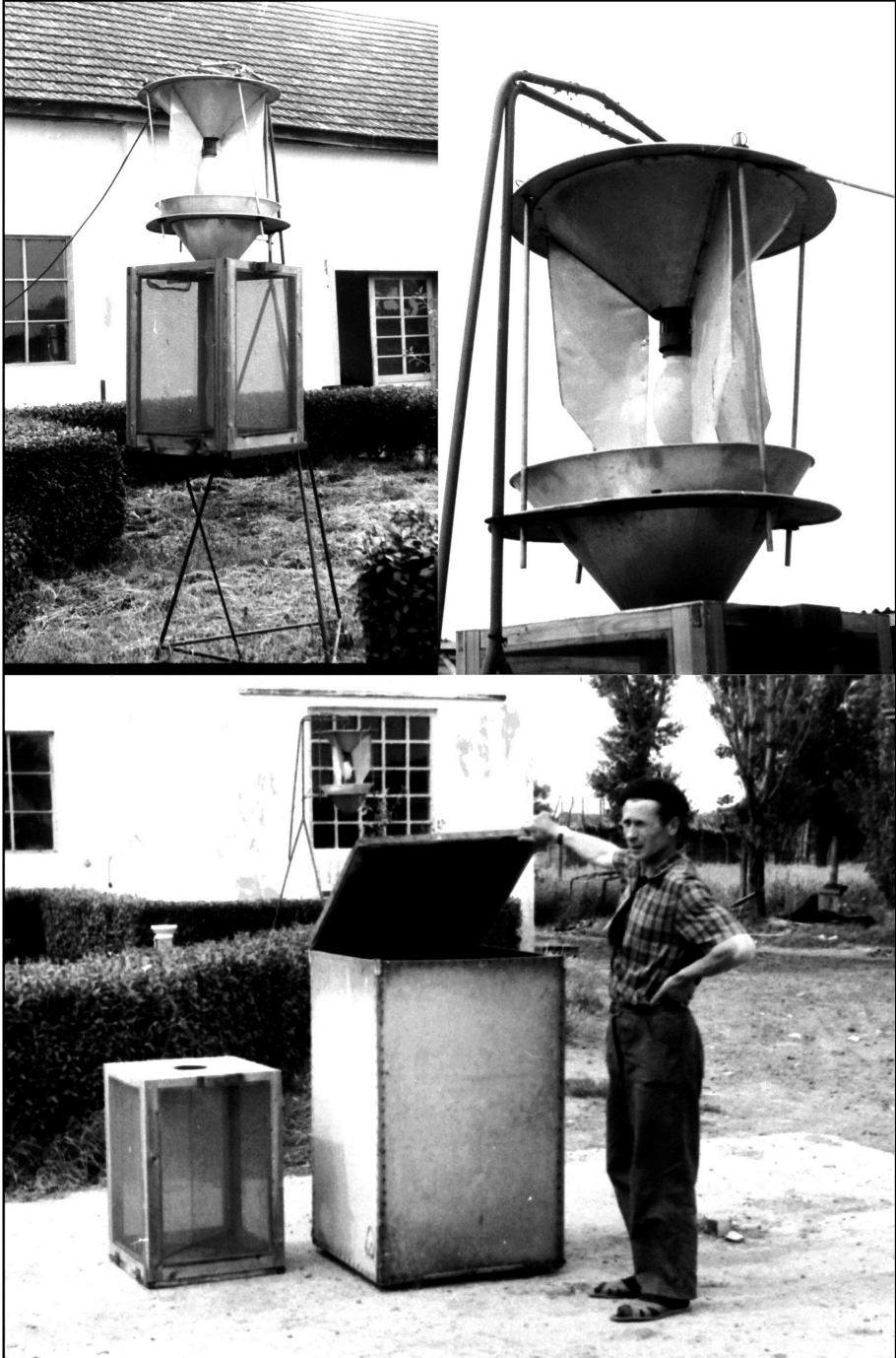
Figure 5. Becse-type light trap in Bečej (Serbia, in 1972)
