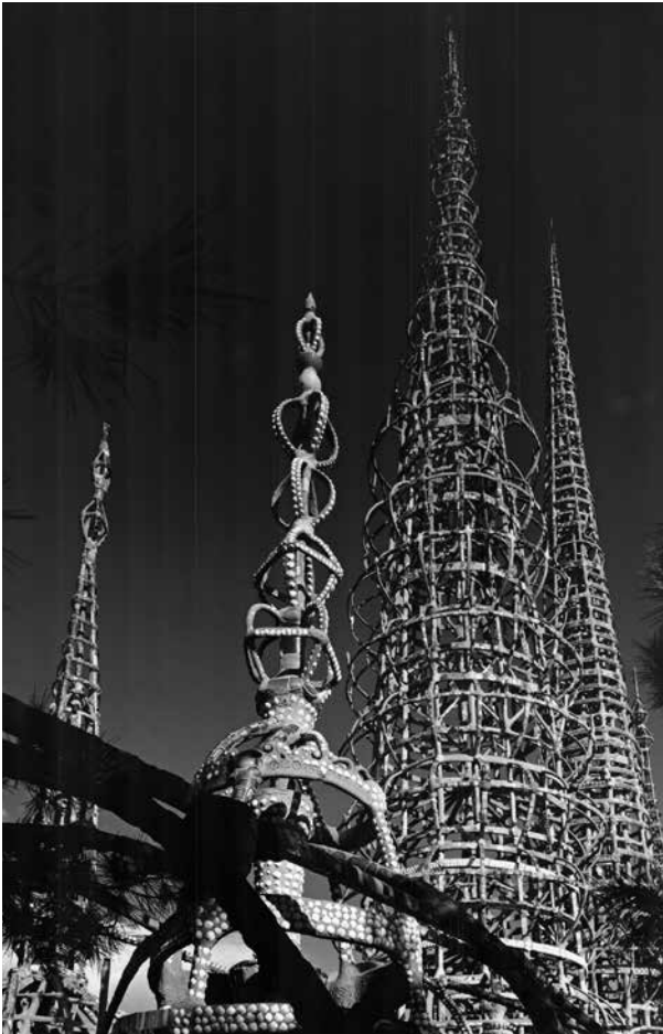
5. Simon Rodia: Watts Towers, Los Angeles, 1966 © Julius Shulman
